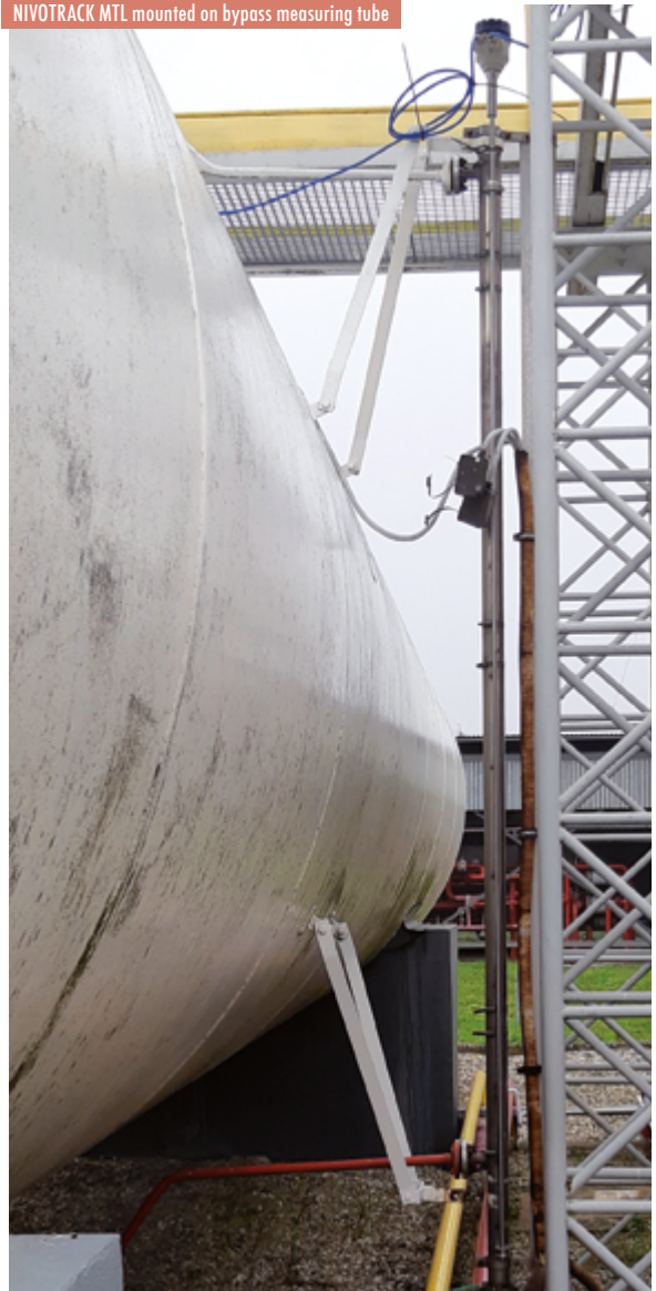
NIVOTRACK MTL mounted on bypass measuring tube
