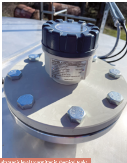
NIVOPOINT magnetic tracking level switch and EchoTREK compact ultrasonic level transmitter in chemical tanks
