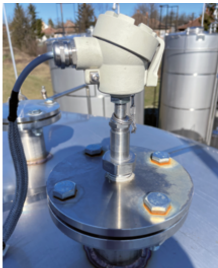
NIVOPOINT magnetic tracking level switch and EchoTREK compact ultrasonic level transmitter in chemical tanks
